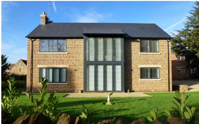
High St – an example of recent development in Ecton
