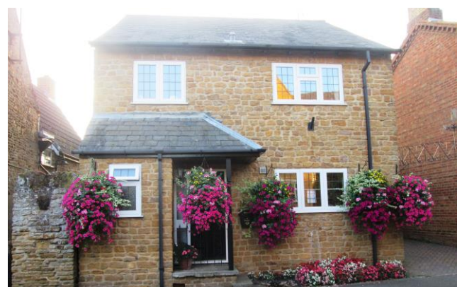
Example of infill development, High St
